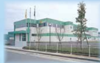
Mie Plant (TA & IT Plant)
